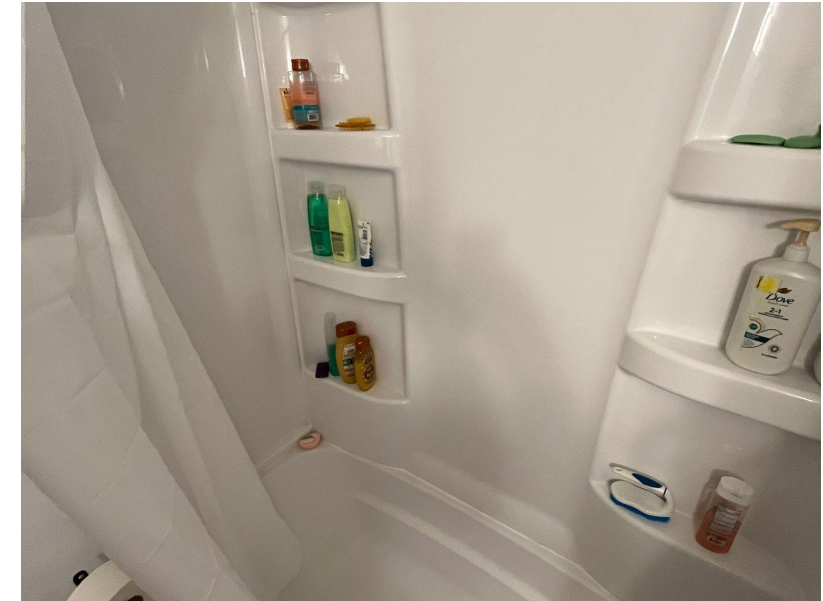
Mold removed, new tub and surround installed.
